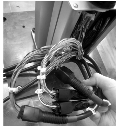
After connecting four cables
